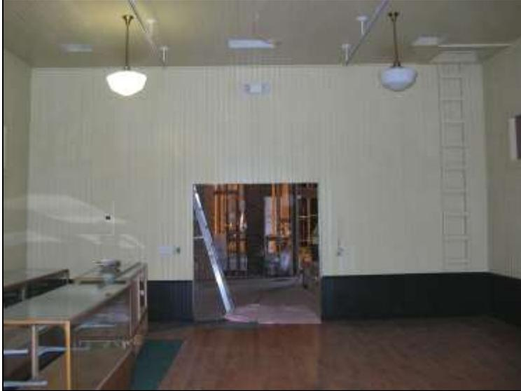
Baggage room south wall with renovated tongue-and-groove wall covering and ceiling, new opening for doorway to visitor center, oak laminate flooring, and light fixtures consistent with the period. The sliding freight door facing the tracks remains operational with original track and rollers. This room now houses the Colfax area museum. Track lights are included to illuminate historic displays.
