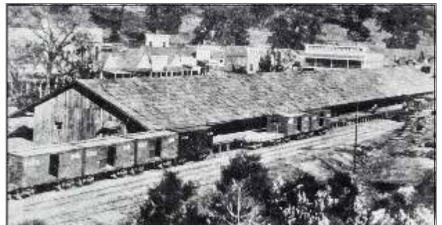
CPRR FREIGHT SHED BUILT IN 1865 ON DOWNTOWN SIDE OF THE TRACKS. MAIN STREET BUILDINGS ARE BEYOND THE SHED. (SIERRA HERITAGE MAGAZINE)
