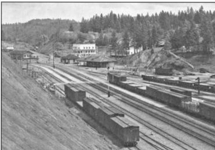
MAY 5, 1915 VIEW FROM HILLSIDE ON SOUTH MAIN STREET. TRACK REALIGNMENT WAS PROGRESSING, WITH NEW TRACKS LAID TO GRASS VALLEY STREET. THE HILLSIDE BEYOND THE FREIGHT DEPOT WAS REMOVED IN 1913-14 TO MAKE ROOM FOR NEW NCNG AND MAINLINE TRACK ALIGNMENT. THE NEVADA COUNTY QUARTZ MONUMENT HAS BEEN RELOCATED, BUT INSTALLATION OF NEW TRACKS THROUGH THE CLEARED AREA WOULD WAIT UNTIL THE FREIGHT DEPOT WAS MOVED LATER IN MAY. (SP COLLECTION, SIGNOR - DONNER PASS)
