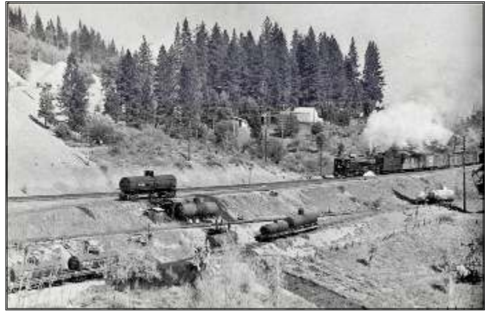
VIEW OF OILVILLE, JUST NORTH OF THE HWY 174 OVERCROSSING. OIL WAS TRANSFERRED FROM SP CARS TO NCNG CARS AND ENGINES ON THE LOWER TRACKS. NOTE THE CAB-FORWARD POWER ON THE SP TRAIN ON THE UPPER TRACK. THE NCNG TURNTABLE WAS TO THE RIGHT OF THIS 1940 SCENE. THE TWILIGHT YEARS OF THE NCNG. (JF OREM PHOTO, SIGNOR – DONNER PASS)
