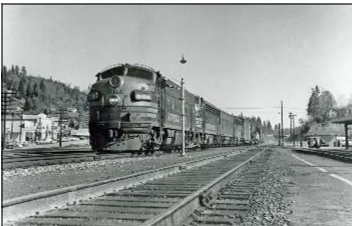
F7 DIESEL ENGINES IN "BLACK WIDOW" PAINT AT COLFAX DEPOT IN 1962. NOTE ENGINE CREW ABOUT TO SNARE TRAIN ORDERS. (BOB MORRIS PHOTO. PSRHS COLLECTION)
