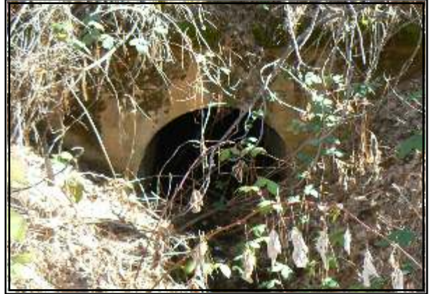
Examples of old and new culvert construction under railroad fills. Photos at left and upper right show both ends of a Rocklin granite rockwork culvert under an original fill near Wirt. Photo at lower right is a concrete culvert under the 1914 fill. Roger Staab photos.
