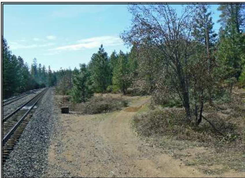
In the photo at left taken near the same location, the old grade can easily be seen veering to the right from the present grade. The fill on the double track in the distance serves both the 1914 second track and the realigned original grade. The power pole near the right edge of the photo is an old square telegraph pole. Roger Staab photo.
