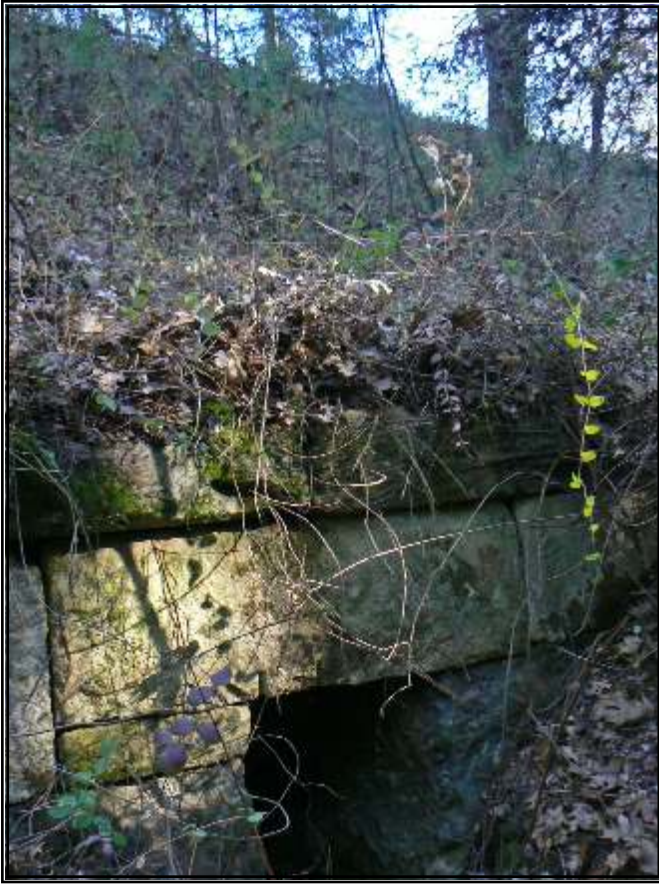
Examples of old and new culvert construction under railroad fills. Photos at left and upper right show both ends of a Rocklin granite rockwork culvert under an original fill near Wirt. Photo at lower right is a concrete culvert under the 1914 fill. Roger Staab photos.
