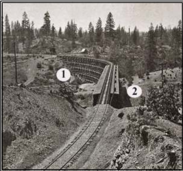
Above, looking westbound, the 1866 curved wooden trestle (1) can be seen beyond the wooden bridge (2) at Long Ravine. The trestle portion was covered with fill in 1876. The circa 1900 photo at upper right shows the curved fill (1) where the trestle once stood, and the steel bridge (2) that replaced the wooden bridge in 1890. At right, an eastbound passenger train with helper is on one of the two Long Ravine Bridges in 1941. Photos above and right courtesy of Jack Duncan. Photo above right from PSRHS collection.
