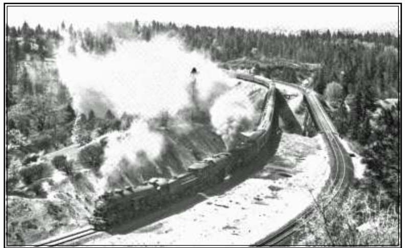
Above, looking westbound, the 1866 curved wooden trestle (1) can be seen beyond the wooden bridge (2) at Long Ravine. The trestle portion was covered with fill in 1876. The circa 1900 photo at upper right shows the curved fill (1) where the trestle once stood, and the steel bridge (2) that replaced the wooden bridge in 1890. At right, an eastbound passenger train with helper is on one of the two Long Ravine Bridges in 1941. Photos above and right courtesy of Jack Duncan. Photo above right from PSRHS collection.
