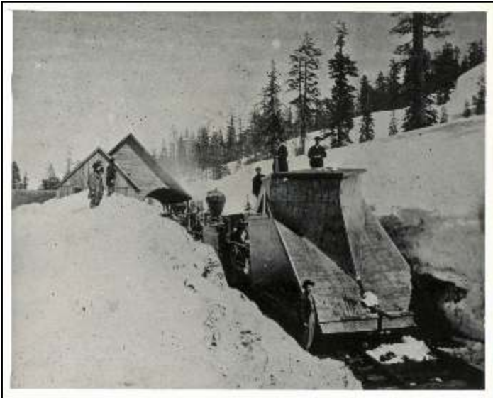
A bucker plow at Cisco. (Ken Yeo Collection) These were pushed through drifted snow by several locomotives, as shown in the lower photo taken at Blue Canyon in 1890. Derailments were a frequent problem. (Lower photo from Best – Snowplow)
