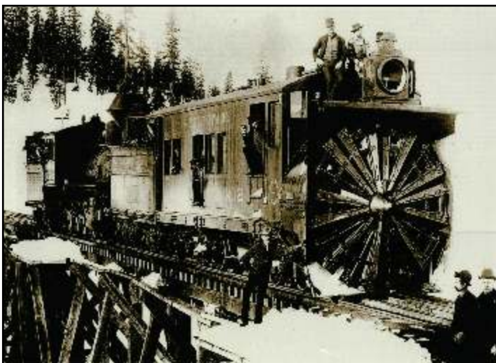
Central Pacific's new Leslie rotary poses at Cascade in 1888. The rotary would prove invaluable in clearing the blockaded tracks in the storms of 1889-90. More rotaries would soon be added to the roster on the Donner route. (PSRHS Collection)
