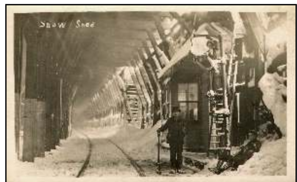
Inside the Snowsheds (Ken Yeo Collection)
