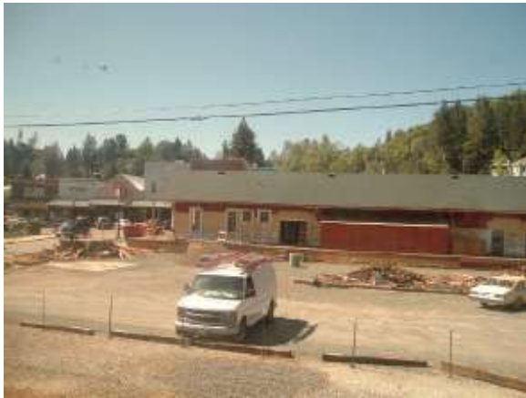
Colfax Freight Depot before repainting, April 1, 2004 (Lyle Brown photo)
