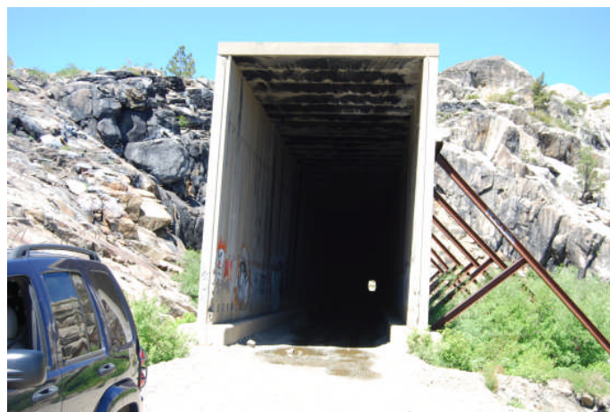
East Portal Tunnel 6
