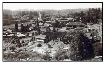
The photo at left shows many of the changes that took place in Colfax during the double-tracking in 1911-15. The mainline tracks were realigned through town, which involved removing two major hillsides. The 9-stall engine house was completed, along with an extensive yard and wye track for turning engines.
