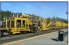
This large trencher removed ballast at each end of the old ties. The TRT-900 then pulled up old ties and placed new concrete ties. *Photos by Roger Staab*
