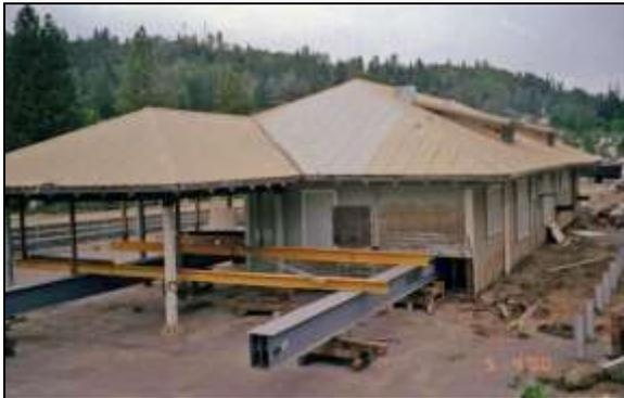
Depot being prepared to be moved aside to pour new slab foundation. *City of Colfax photo.*
