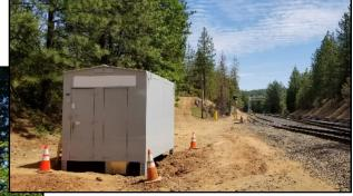
As of 5/11, the signals are up on the cantilever signal bridges at Gold Run. The signal bungalow has been placed, but no trenching activity to the power switches yet.
