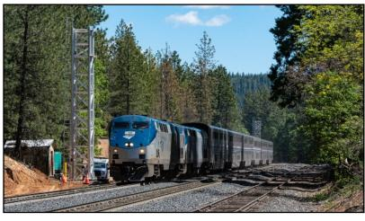
By 4/30/2020 when the photo at left was taken, UP had installed the second support truss for the west cantilever signal bridge. Amtrak No. 5 passes through the area with both cantilever supports visible.
