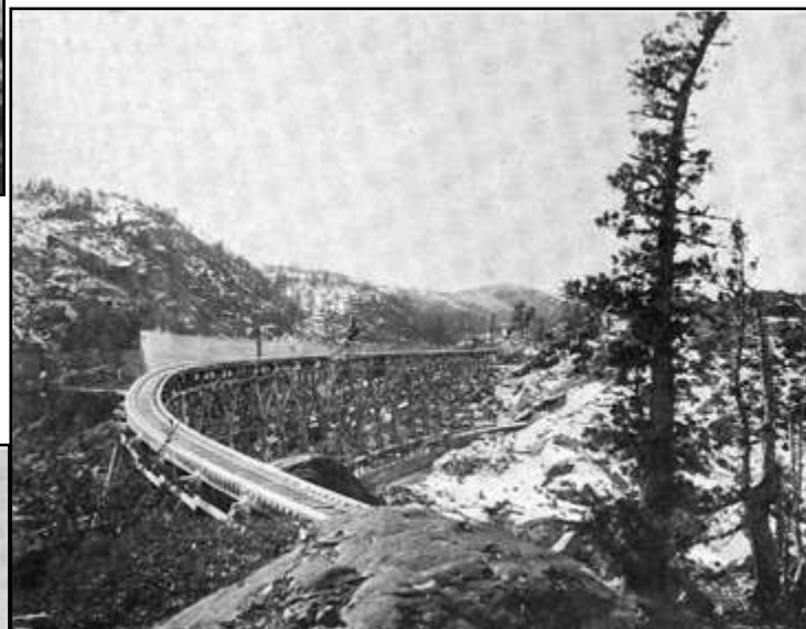
This view shows the 500 foot long narrow gauge curved wood trestle looking back toward the main dam. The new spillway was constructed in the depression crossed by the trestle.
