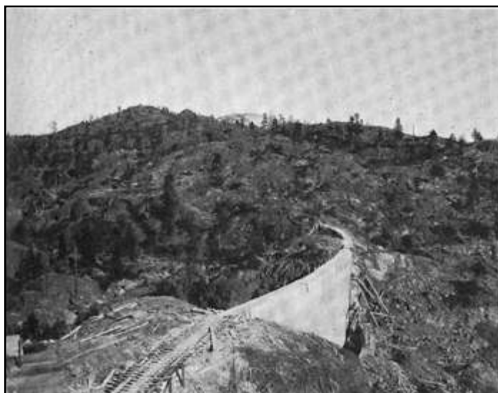
At the far end of the 3000 foot narrow gauge railroad three secondary dams were built to block low areas that were breached by the new reservoir height. Dam #3 increased the height of the old spillway. New dams 4 and 5 shown in this image were separated slightly by a ridge. When the main dam was raised to 275 feet in 1919, these two secondary dams became one.
