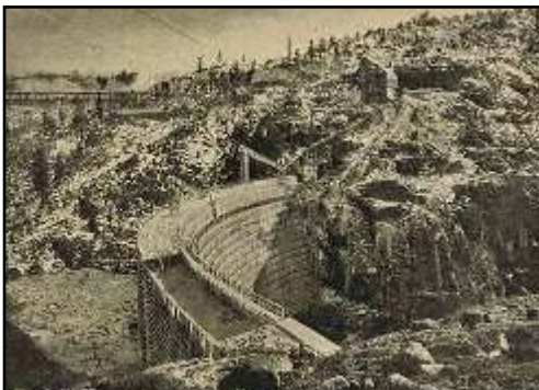
Spaulding Dam nearing 225 feet high. The batch plant is at upper right. Conveyors on the dam distributed the concrete to desired pour locations.
