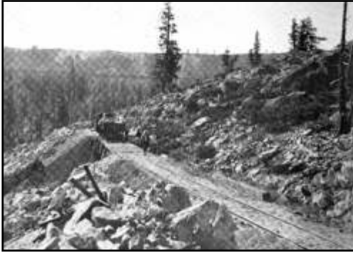
At left is a portion of the standard gauge spur being built by PG&E to deliver equipment and materials to the dam construction site. At right is the narrow gauge Shay purchased from Birce and Smart and used by PG&E for moving supplies and clearing timber from the area to be flooded by the dam.
