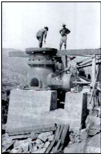
The PG&E standard gauge spur was used to move large rock crushers (left) and huge check valves (right) to the construction site, as well as carloads of gravel & cement.
