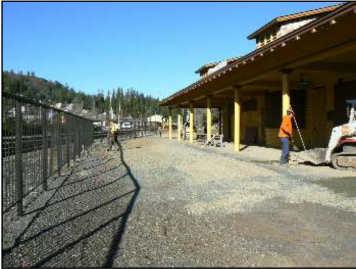
Contractor performing grading and asphalt installation in the area surrounding the depot.
