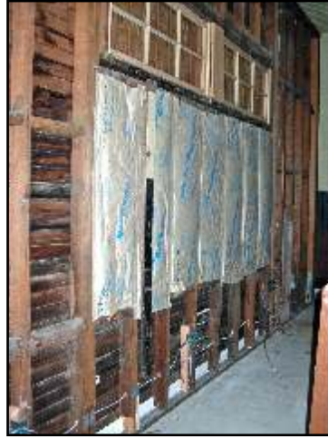
In the photos above, the north wall of the baggage room required the addition of a section of plywood sheer wall to meet earthquake standards. The beaded tongue-and-groove boards were removed from the entire wall and insulation added along with shear plywood at far right corner and nailing strips.
