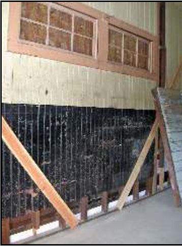
In the photos above, the north wall of the baggage room required the addition of a section of plywood sheer wall to meet earthquake standards. The beaded tongue-and-groove boards were removed from the entire wall and insulation added along with shear plywood at far right corner and nailing strips.
