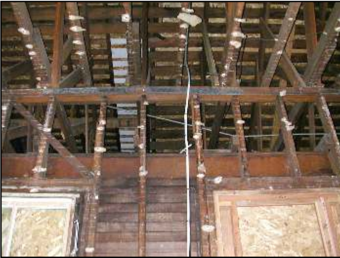
At left, residue from old plaster and sheetrock wall and ceiling coverings had to be removed from framing members by volunteers before new work could begin. At right, volunteers researched, procured and installed new roof signs for Colfax station consistent with historical signage..
