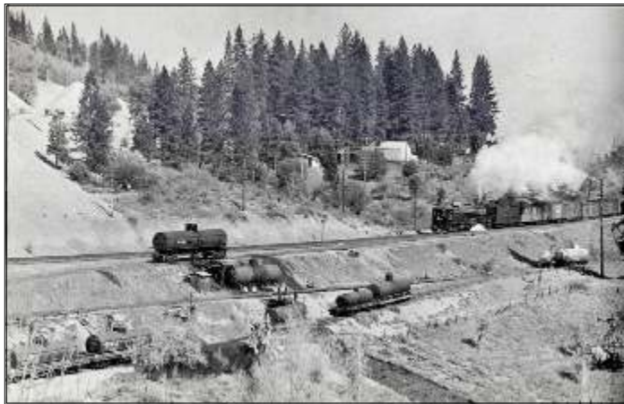
VIEW OF OILVILLE, JUST NORTH OF THE HWY 174 OVERCROSSING. OIL WAS TRANSFERRED FROM SOUTHERN PACIFIC CARS TO NCNG EQUIPMENT ON THE LOWER TRACKS. NOTE THE CAB-FORWARD POWER ON THE SOUTHERN PACIFIC TRAIN ON THE UPPER TRACK. THE NCNG TURNTABLE WAS TO THE RIGHT OF THIS 1940 SCENE. CAPTURED DURING THE TWILIGHT YEARS OF THE NCNG. (J.F. OREM PHOTO. SIGNOR - DONNER PASS)
