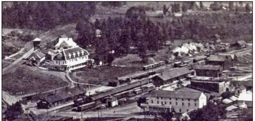
IN THIS CIRCA 1904 VIEW, THE LARGE BUILDING TO THE LEFT IS THE GILLEN (COLFAX) HOTEL, BUILT IN 1903. BELOW IT IS THE 1865 PASSENGER DEPOT, WHICH BURNED IN 1905. TO THE RIGHT OF THE PASSENGER DEPOT ARE THE NCNG TRANSFER SHED AND FREIGHT DEPOT. DOWNTOWN BUILDINGS ARE AT BOTTOM RIGHT. NCNG TRAINS ARRIVED ON THE FAR SIDE OF THE PASSENGER DEPOT. THE FREIGHT DEPOT AND TRANSFER SHED WERE SOON MOVED ACROSS THE MAINLINE TRACKS, AND A NEW PASSENGER DEPOT CONSTRUCTED. (PSRHS COLLECTION)
