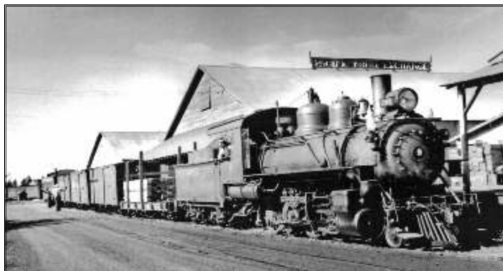
NCNG ENGINE #9 ON RAILROAD AVENUE NEXT TO THE PACIFIC FRUIT EXCHANGE FRUIT SHEDS IN 1939. NARROW GAUGE TRACKS RAN ALONG TODAY'S RAILROAD AVENUE. (AL PHELPS PHOTO)
