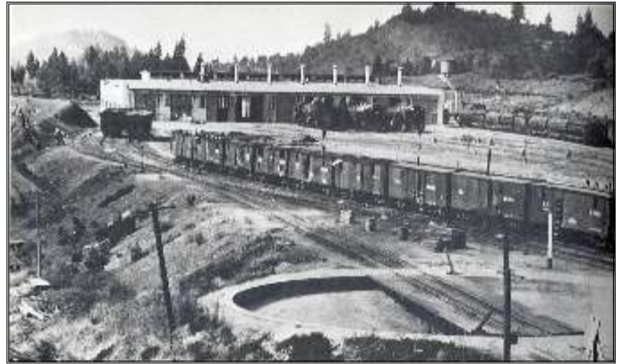
BELOW, CIRCA 1913: THE ENGINE HOUSE IS IN THE BACKGROUND AND 65-FOOT TURNTABLE IN THE FOREGROUND LOOKING SOUTHWEST FROM TODAY'S INTERSECTION OF RAILROAD AVE. AND OAK ST. THE TURNTABLE WAS ABANDONED AFTER THE WYE TRACK NEAR THE ENGINE HOUSE WAS COMPLETED. THE TRACKS IN THE FOREGROUND LINED WITH RAILCARS WERE PART OF THE ORIGINAL CPRR ALIGNMENT. (ALAN ASKE, SIGNOR - DONNER PASS)
