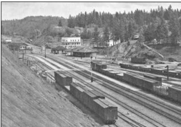
MAY 5, 1915 VIEW FROM HILLSIDE ON SOUTH MAIN STREET. TRACK REALIGNMENT WAS PROGRESSING, WITH NEW TRACKS LAID TO GRASS VALLEY STREET. THE HILLSIDE BEYOND THE FREIGHT DEPOT WAS REMOVED IN 1913-14 TO MAKE ROOM FOR NEW NCNG AND MAINLINE TRACK ALIGNMENT. THE NEVADA COUNTY QUARTZ MONUMENT HAS BEEN RELOCATED. BUT INSTALLATION OF NEW TRACKS THROUGH THE CLEARED AREA WOULD WAIT UNTIL THE FREIGHT DEPOT WAS MOVED LATER IN MAY. (SP COLLECTION, SIGNOR – DONNER PASS)
