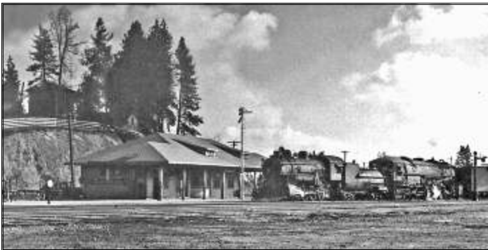
COLFAX-BASED CONSOLIDATION HELPER AT THE HEAD END OF A CAB-FORWARD-POWERED FRUIT TRAIN BY THE COLFAX DEPOT IN 1940. NOTE WATER COLUMN AT FAR RIGHT AND TRAIN ORDER SEMAPHORE BY THE DEPOT. (JF. OREM PHOTO, SIGNOR - DONNER PASS)
