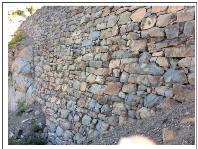
Detail of China Wall with hand laid stone without mortar. The track above operated from 1868 until 1993, carrying heavy modern trains without movement or damage to the wall.
