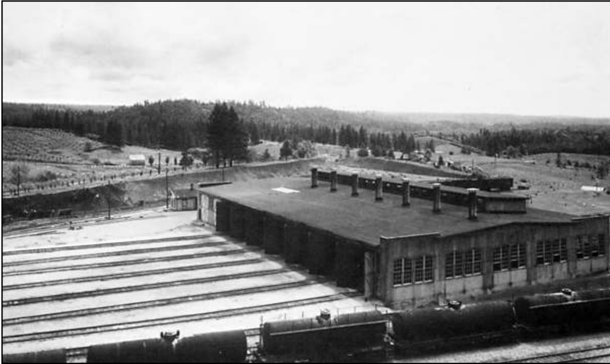
1912 Engine House with Wye Track Beyond It
