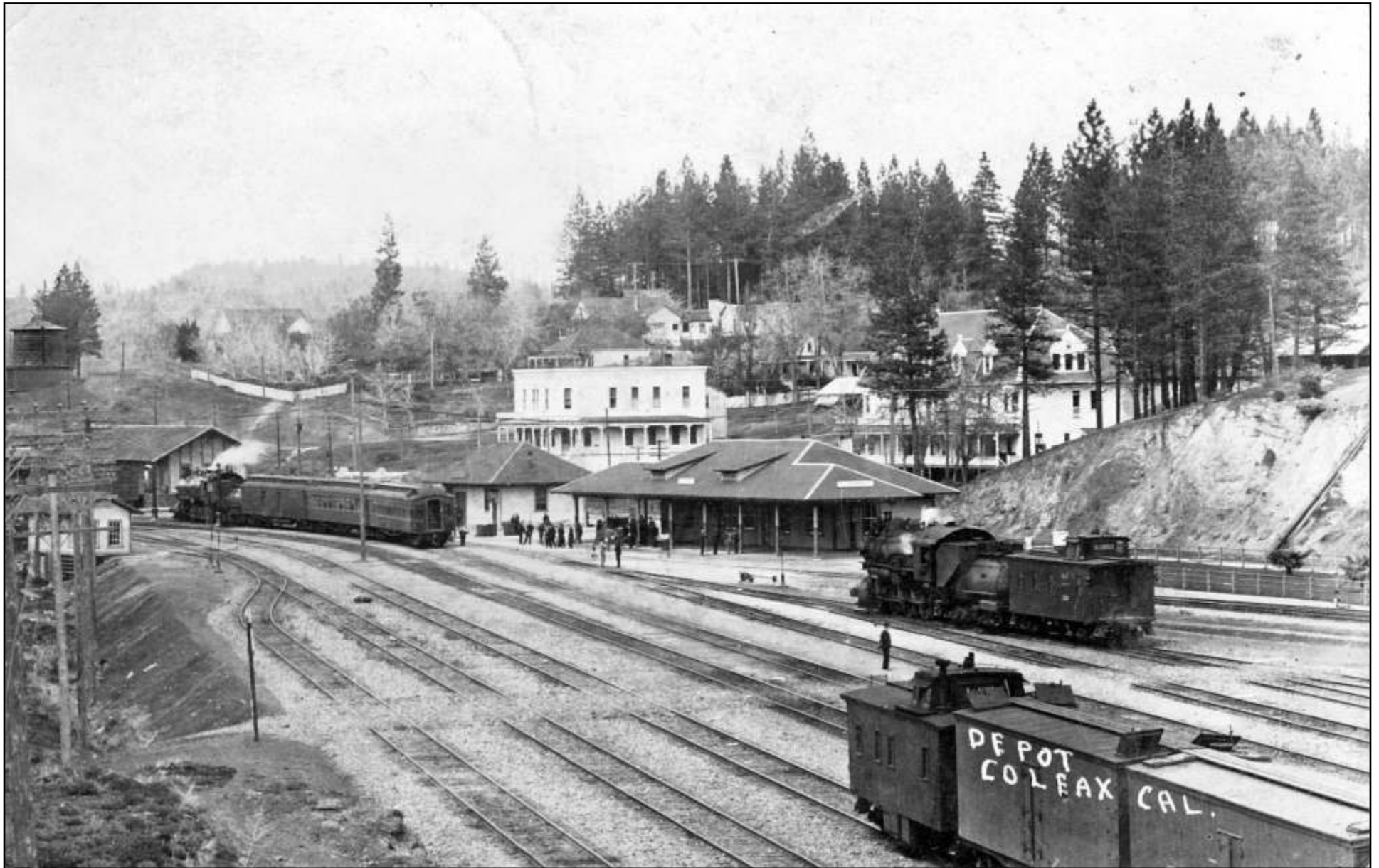
1912 - Double Tracking Underway. Fill and New Yard Tracks Extend Beyond Passenger Depot, then Curve to Old Alignment Going Past Freight Depot
